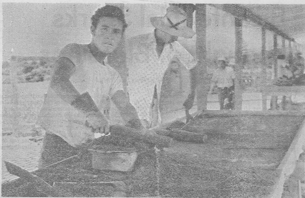
Guatemalan workers pound mix of materials into molds to produce building blocks.
